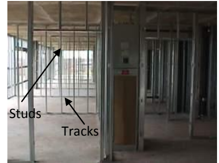
IMAGE 6-4: Tracks and Steel Studs
