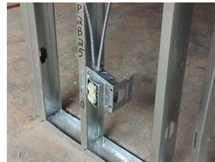
IMAGE 6-5: Electrical conduits/Receptacle
